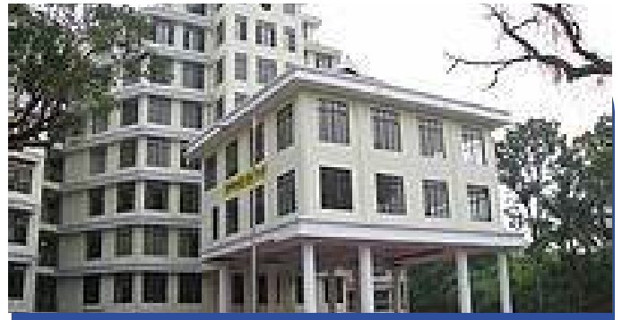
Collectorate Trivandrum - 3.2 km
